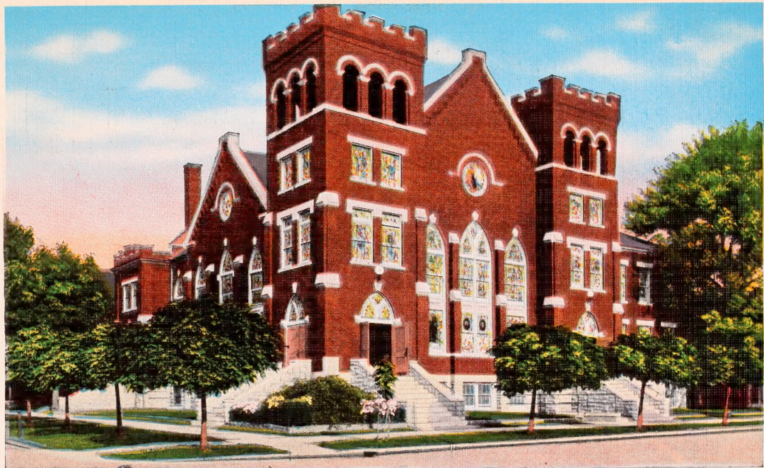
FIRST METHODIST EPISCOPAL CHURCH, PARSONS, KANSAS—22
